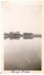
1938 Hurricane - Reef Road (FF_Hurricane1938_F1_018)
