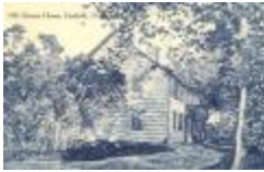
Old Benson House, Fairfield, Conn. (PC_FF_Houses_Benson_02)
