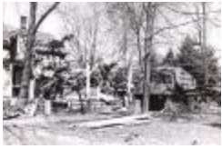
Hurricane of 1954-Clearing Rubble (FF_Hurricane1954_001)
