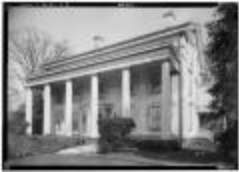
739 Old Post Road (FF_BLDGS_739Old Post Rd_2)
