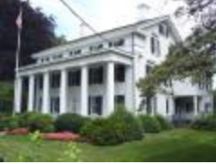
739 Old Post Road (FF_BLDGS_739Old Post Rd_9)
