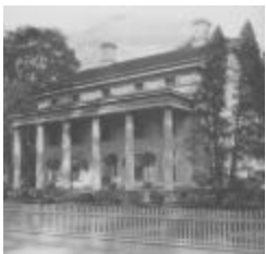
739 Old Post Road (FF_BLDGS_739Old Post Rd_12)
