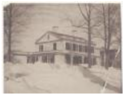
480 Old Post Road (FF_BLDGS_480Old Post Rd_3)
