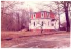
808 Old Post Road (FF_BLDGS_808Old Post Rd_5)
