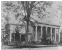
458 Old Post Road (FF_BLDGS_458Old Post Rd_1)
