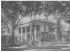
458 Old Post Road (FF_BLDGS_458Old Post Rd_4)
