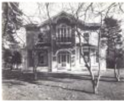
415 Old Post Road (FF_BLDGS_415Old Post Rd_3)
