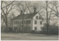
543 Old Post Road (FF_BLDGS_543Old Post Rd_2)
