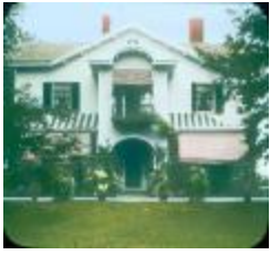
Jennings House (MOW_137_Jennings House)
