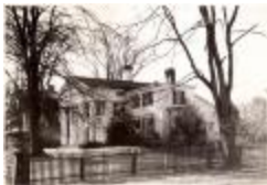
536 Old Post Road (FF_BLDGS_536Old Post Rd_2)
