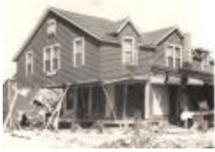
Hurricane 1938 Fairfield Beach house porch destroyed (FF_Hurricane1938_F1_021)
