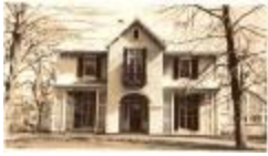
363 Old Post Road (FF_BLDGS_363Old Post Rd_2)
