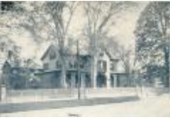
766 Old Post Road (FF_BLDGS_766Old Post Rd_2)
