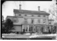
739 Old Post Road (FF_BLDGS_739Old Post Rd_3)
