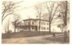
85 Old Post Road (FF_BLDGS_85Old Post Rd_2)
