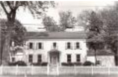
766 Old Post Road (FF_BLDGS_766Old Post Rd_3)
