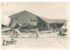
1938 Hurricane Collapsed Home at Beach (FF_Hurricane1938_F1_016)
