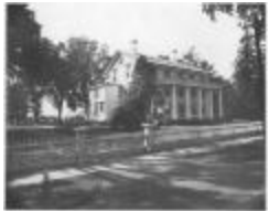
739 Old Post Road (FF_BLDGS_739Old Post Rd_10)
