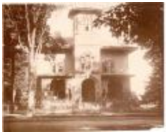
432 Old Post Road (FF_BLDGS_432Old Post Rd_1)
