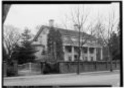
739 Old Post Road (FF_BLDGS_739Old Post Rd_1)
