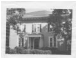
432 Old Post Road (FF_BLDGS_432Old Post Rd_2)
