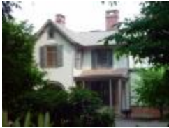
363 Old Post Road (FF_BLDGS_363Old Post Rd_3)
