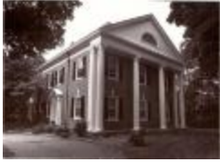
388 Old Post Road (FF_BLDGS_388Old Post Rd_1)
