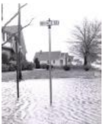
Quincy Street 1953 Hurricane (FF_Hurricane1953_F1_005)
