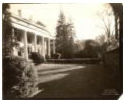
739 Old Post Road (FF_BLDGS_739Old Post Rd_18)
