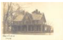
690 Old Post Road (PC_FF_Houses_690 Old Post Rd)
