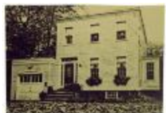
126 Old Post Road (FF_BLDGS_126Old Post Rd_1)
