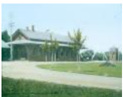
Fairfield Railroad Station (MOW_154_Fairfield Railroad Station)
