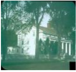
Burr Homestead (MOW_133a_Burr Homestead-wall)
