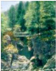
Tree Bridge from the North (MOW_055_Tree Bridge from the North)
