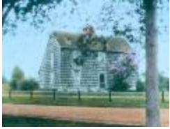
Ogden House (MOW_111_Ogden House)
