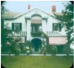
Jennings House (MOW_137_Jennings House)
